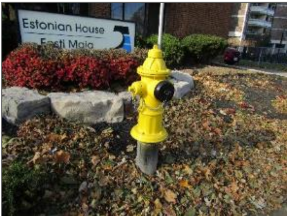
View of the fire hydrant noted at the east portion of the Site.
