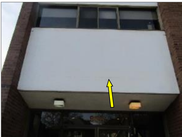
View of the cracks in the cement parking noted on the east elevation of the Phase 3 portion of the Site Building.
