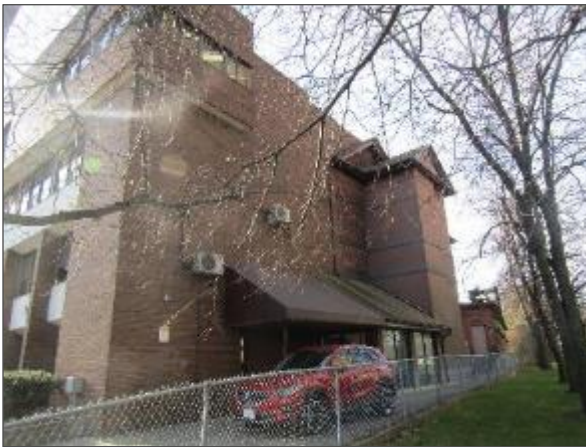
General view of the north elevation of the Site Building.
