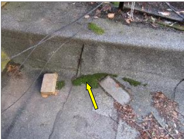
View of moss growth noted at the northeast portion of the modified bitumen roof system serving the Phase 2 portion of the Site Building.
