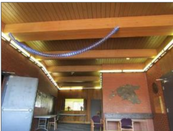
General view of the interior finishes noted within the Grand Hall foyer in the Phase 2 portion of the Site Building.
