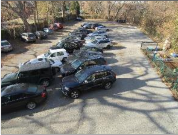
General view of the asphalt paved parking area located at the west portion of the Site.
